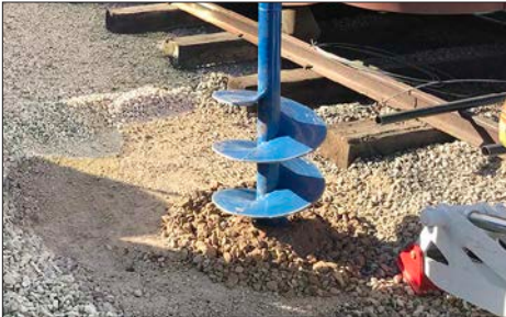
boring the hole
