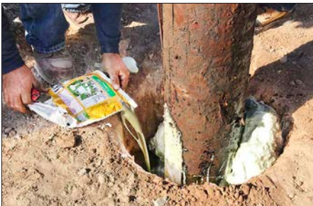
pouring the PostFix foam (Sika PostFix, available in hardware stores, sets way faster than concrete)
