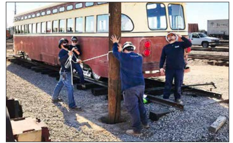
placing the pole
