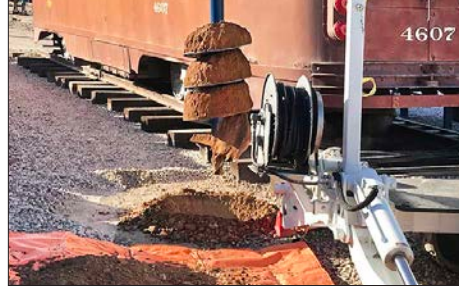
lifting the dirt
