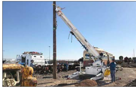
raising the pole
