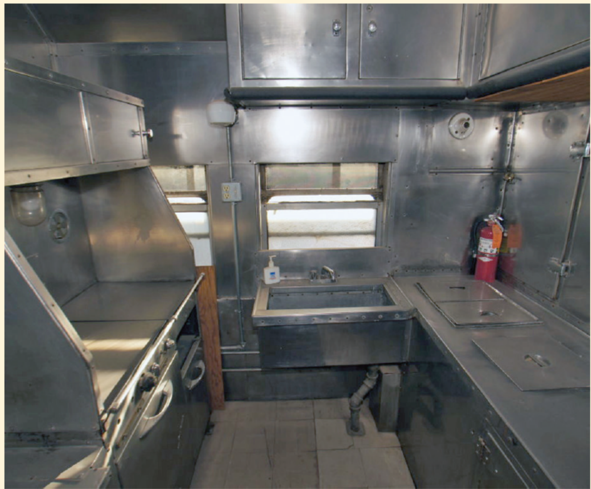
ABOVE: View of kitchen from corridor of Southern 16. Not shown on the drawing is the relocation of the sink to under the window, allowing for more storage and counter space.
